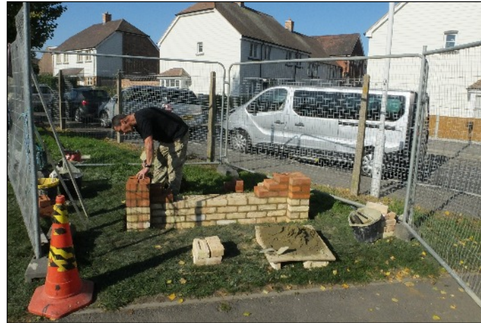
Jon the bricklayer taking great care over building the wall - 16th October 2018
